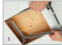
Insert Flex-Z Fast™ installation bracket
