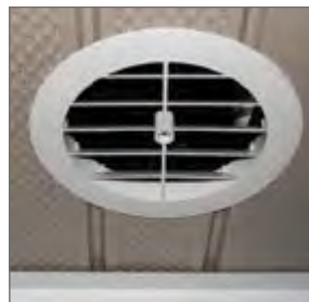
EZ Soffit Vent installed
